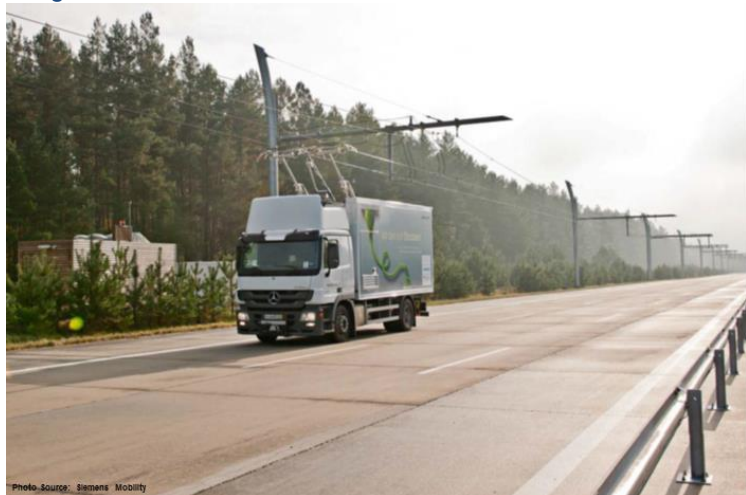
Figure 2: Proposed Catenary System for I-710 Zero-Emissions Corridor (Source: Siemens Mobility).
