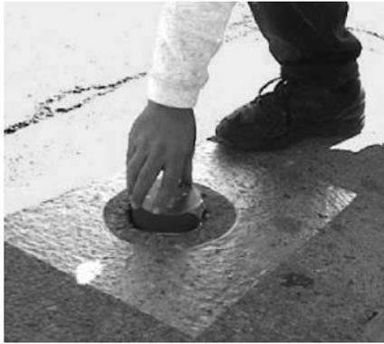
Figure 8. Seattle Center In-surface, Wireless Vehicle Detector
