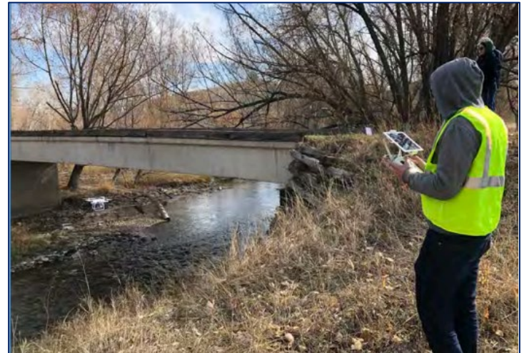
Figure 2: Assessing and Monitoring Bridge Conditions Using UAV (Source: Colorado State University).
