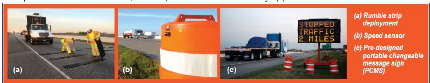
Figure 8: Image showing the components of the end-of-queue warning system including rumble strips, speed sensors and a pre-designed portable changeable message sign (Source: Texas DOT)
