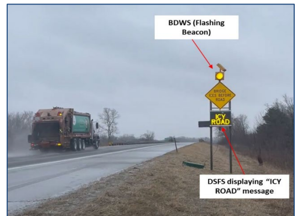
Figure 1: An Activated Bridge Deck Warning System (Source: MDOT)
