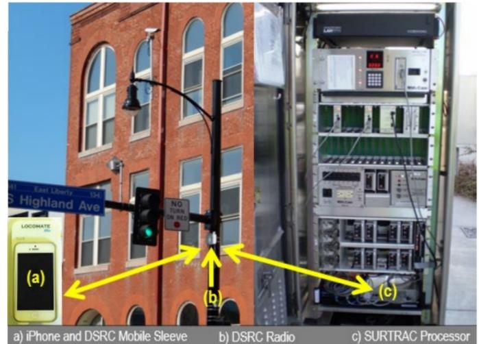
Figure 1. Multiple ITS components enable the safe intersection crossing app. Source: USDOT
